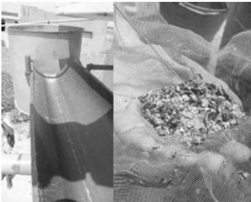
*Contamination can be avoided by frequently cleaning gutters, inlet pipes and collection inlet canals.*
